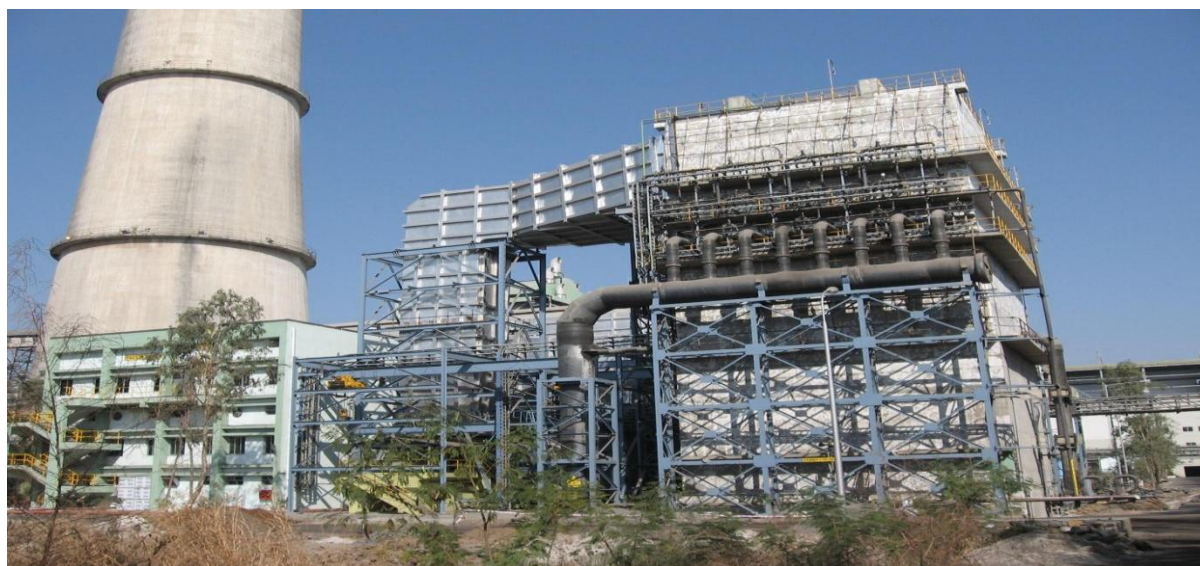
(India's first Sea water FGD system with 100% of flue gas, for 2 X 250 MW Dahanu Thermal Power Station at Dahanu, Maharashtra, India installed by Ducon)
